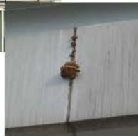
FUNGAL GROWTH DUE TO IMPROPER SEALANT USE
