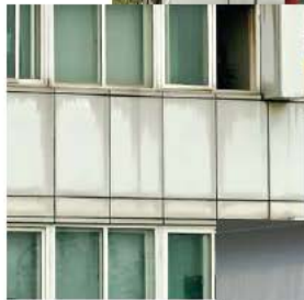
FUNGAL GROWTH DUE TO IMPROPER SEALANT USE
